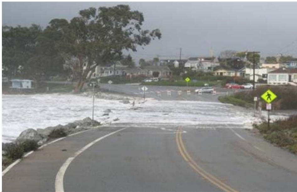
Figure 11. Flooding of a coastal road in Santa Cruz, California
